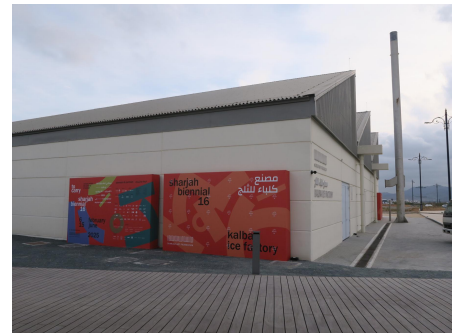
Kalba Ice Factory, Sharjah, United Arab Emirates, February 2025. Photo: Contemporary HUM.
