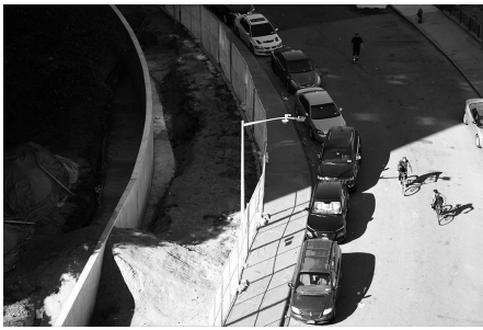
Amy Howden-Chapman, The Walling World (2019). A newly concrete wall erected around NYCHA's Baruch Houses in Manhattan's Two Bridges neighborhood. Construction crews have installed a dirt ramp in order to access both sides of wall designed to stop flooding and storm surges from the nearby East River. Image courtesy the artist.
